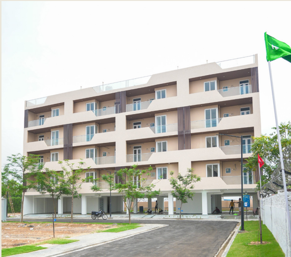
SHF Floors- Exterior
